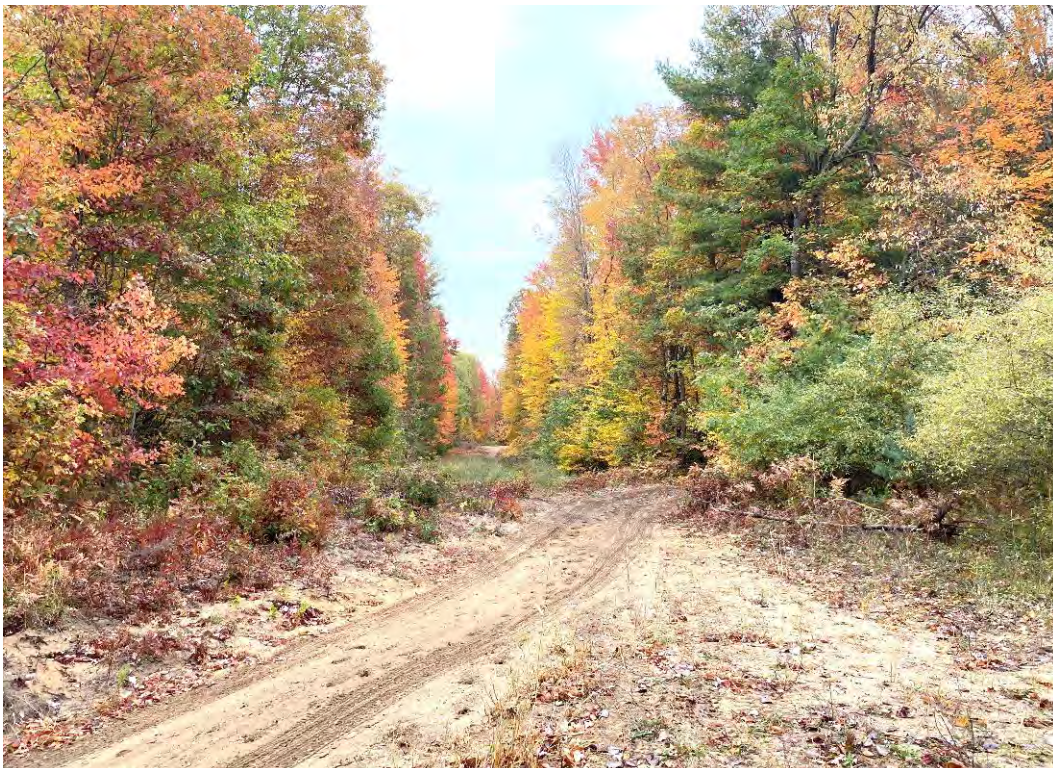
Photo 16: Utility corridor, southern project area, facing east.
